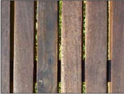
Timber prior to cleaning
